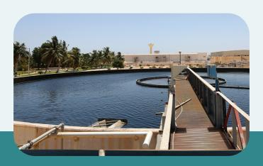
DISC produce treated water at Raysut plant (tertiary treatment plant) where wastewater goes through many chemical and biological stages of treatment till it reaches the required degree of purity according to the international standards.
